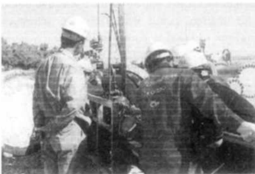
Photo 2 Removing the PIG from the Receiver
